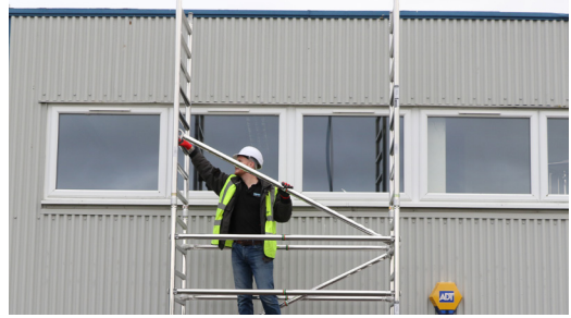
14. Continue erecting the tower fitting the frames and diagonal braces as illustrated using all components. Platforms inserted every 2m complete with handrails. Braces run in a continuous pattern on opposite sides except where interrupted by a platform. Then braces can be stepped up/down 1 rung.
