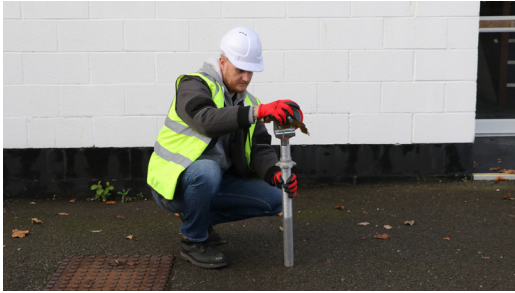
1. Insert castor wheels into adjustable legs
