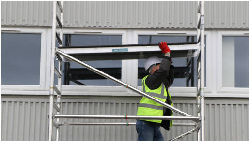
15. For your working platform fit trapdoor on the 6th rung down from the top of the tower.
