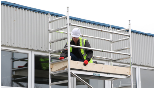
17. Fit toe-boards in correct position
