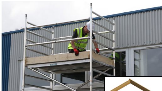
18. Correctly fit toe-boards as shown in the images.
